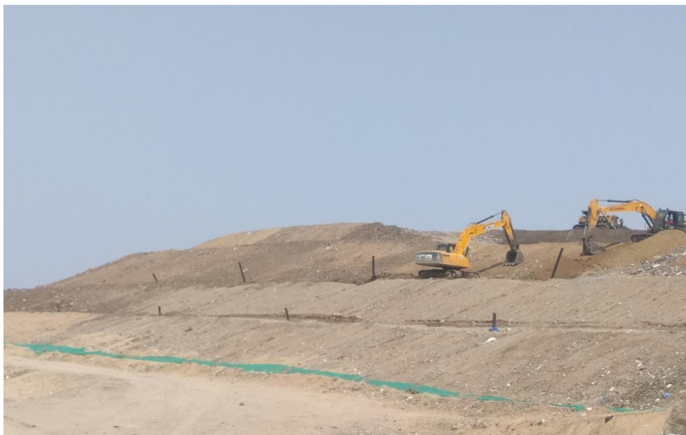
Soil cover on landfill
