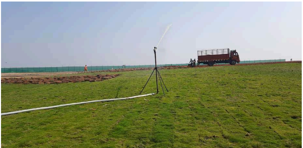
Permeate used for watering green cover on top of capped dump
