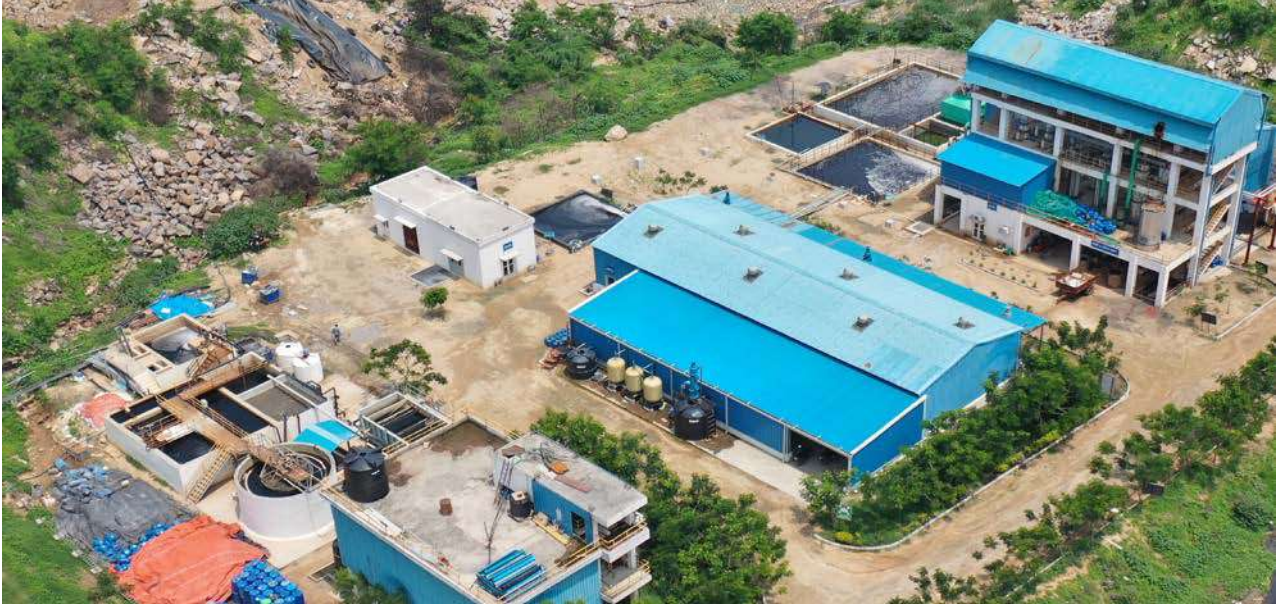
Waste Water Complex: Pretreatment, RO shed, MEE-ATFD system (left to right)
