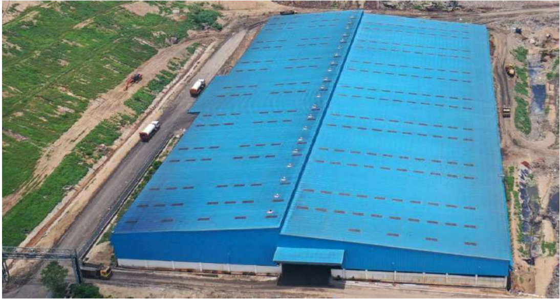
Closed Tipping floor
