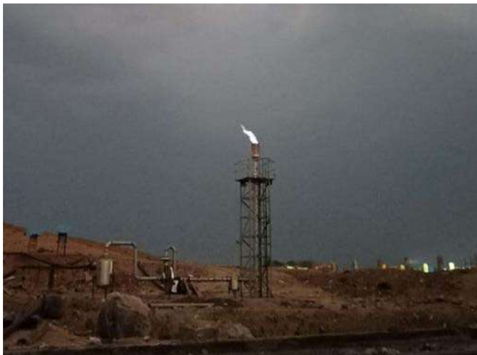
Flaring of excess landfill gas from capped dump
