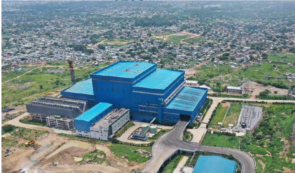
24 MW WTE plant at Jawaharnagar
